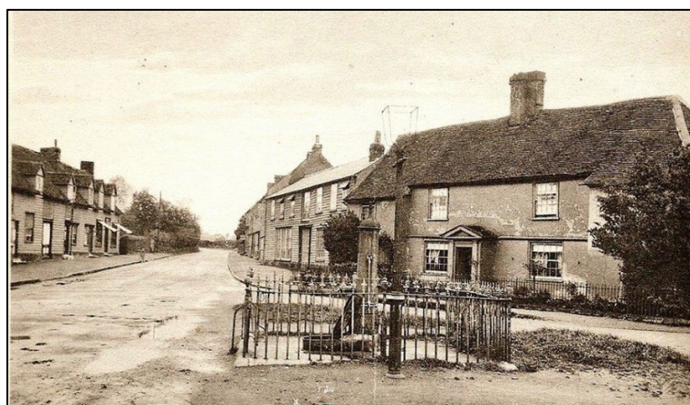
Figure 6: Hooks (later the Pump House)
